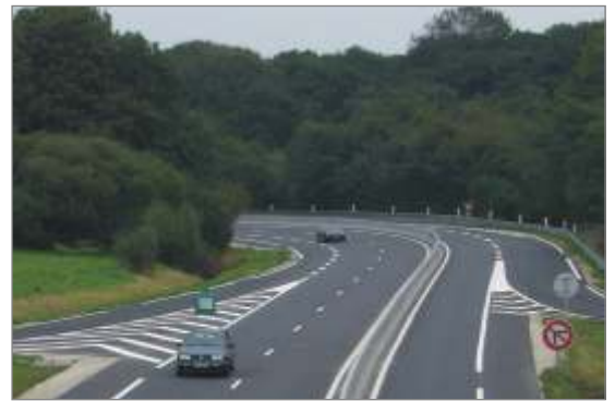
Site after the roadworks
