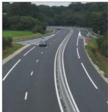
Section with bends after the works
