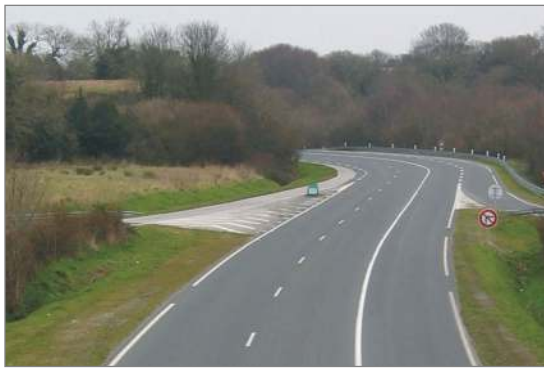
Site before the roadworks
