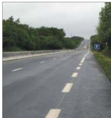
Straight section after the works
