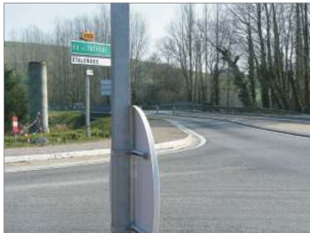
Obstructions to drivers' visibility towards Le Tréport
