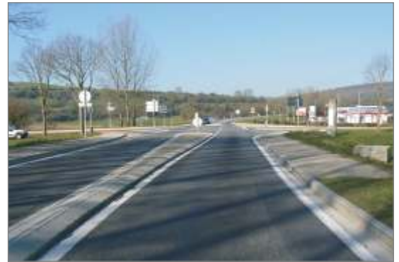
Site after the roadworks
