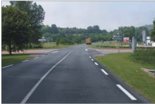
Site before the roadworks
