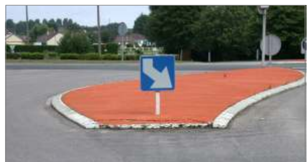
RD226 road coming from Touffreville-sur-Eu Truncated island used to perform left turns via the right
