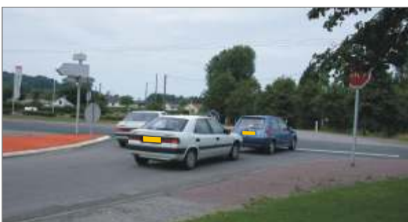
RD226 road coming from Touffreville-sur-Eu Two cars can lay abreast at the stop line
